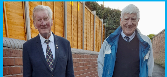
Your local Town Cllrs, who have lobbied the Wyre Forest District Council for some time, welcome the renovation works which have been carried out on the historic wall in Engine Lane. It was in danger of falling down.
