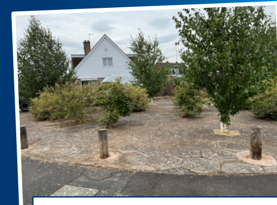
Beechfield Drive, tidy, after the works were carried out for residents.
