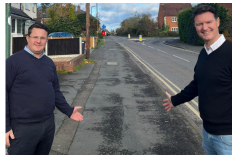
Now work starts to get Hoo Road Pavement resurfaced for pedestrians
