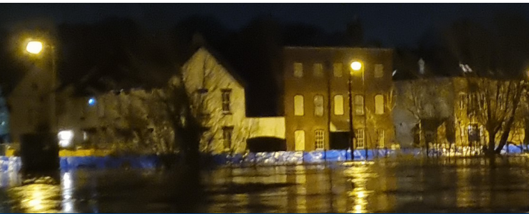
The plans for the permanent flood defences for the Eastern Bank are on schedule for Autumn 2024
