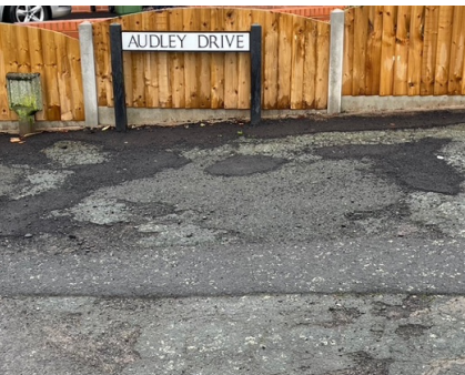
The footpath has been patched and will be fully resurfaced
