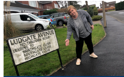
Ludgate Avenue pavement resurfacing completed
