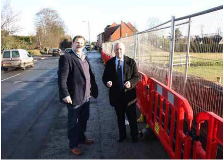
Picture shows Gordon Yarranton and Andrew Tromans by the wall on the Kidderminster Road at Wribbenhall
